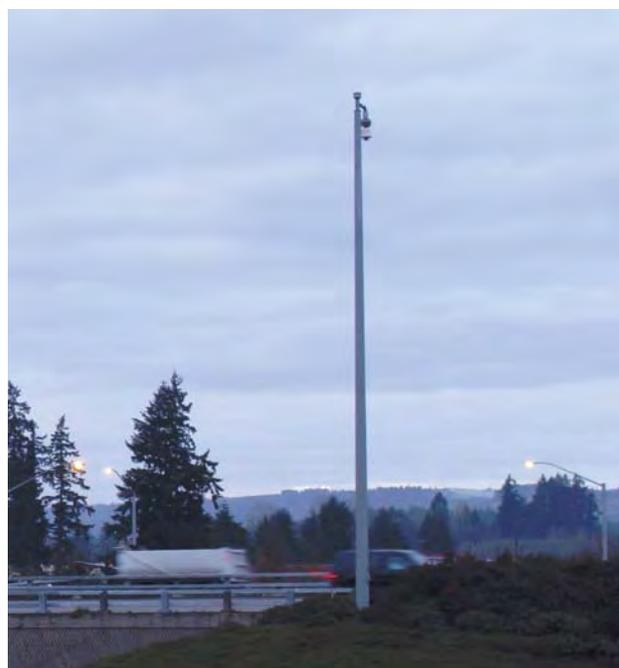
*The CCTV camera mounted above the I-5/Wilsonville Road interchange provides a real-time video feed that allows ODOT to monitor and collect traffic information. The video feed is also available to all transportation users on ODOT’s Trip Check website.*
