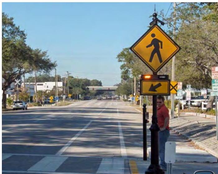
Rectangular rapid flashing beacons at a trail/roadway crossing.
