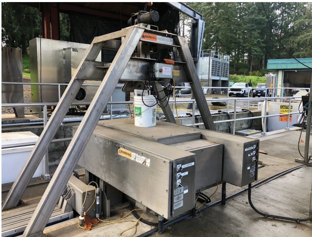
Figure 2-1. Existing TrojanUV4000 system
