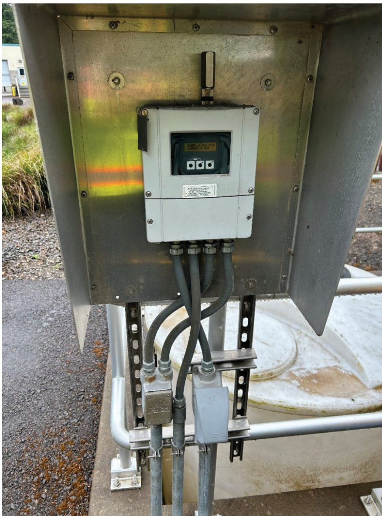
Figure 3-7. Flow meter display
