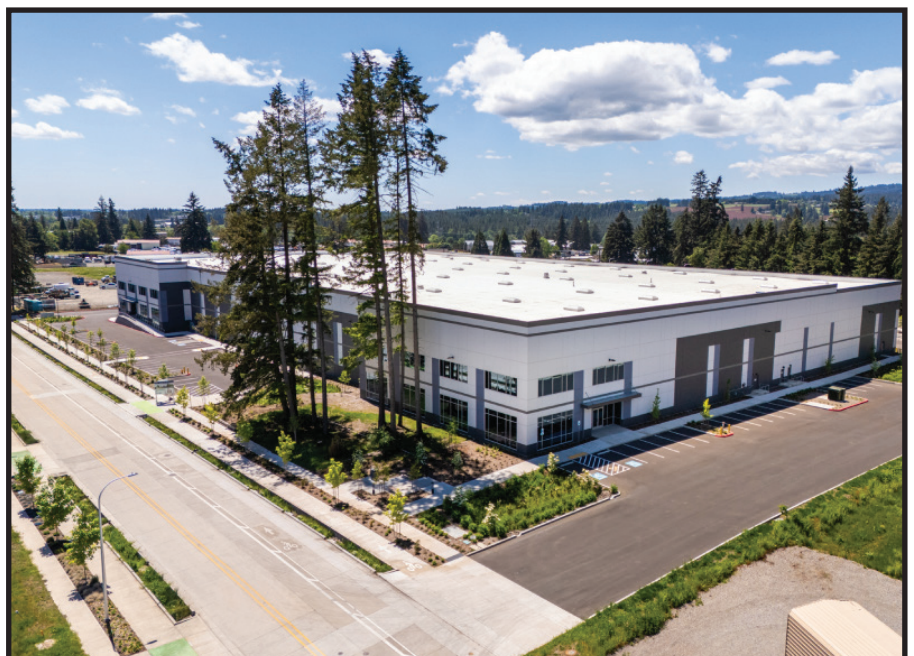
Grahams Ferry Industrial Center, made possible by construction of Garden Acres Road (as shown) as part of the Coffee Creek Urban Renewal Area.
