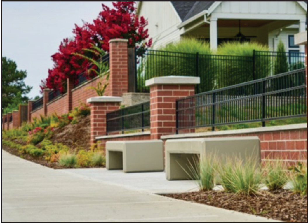
Sidewalk and Bench Installation at Meridian Creek Crossing at Boeckman Road (CIP #4205).
