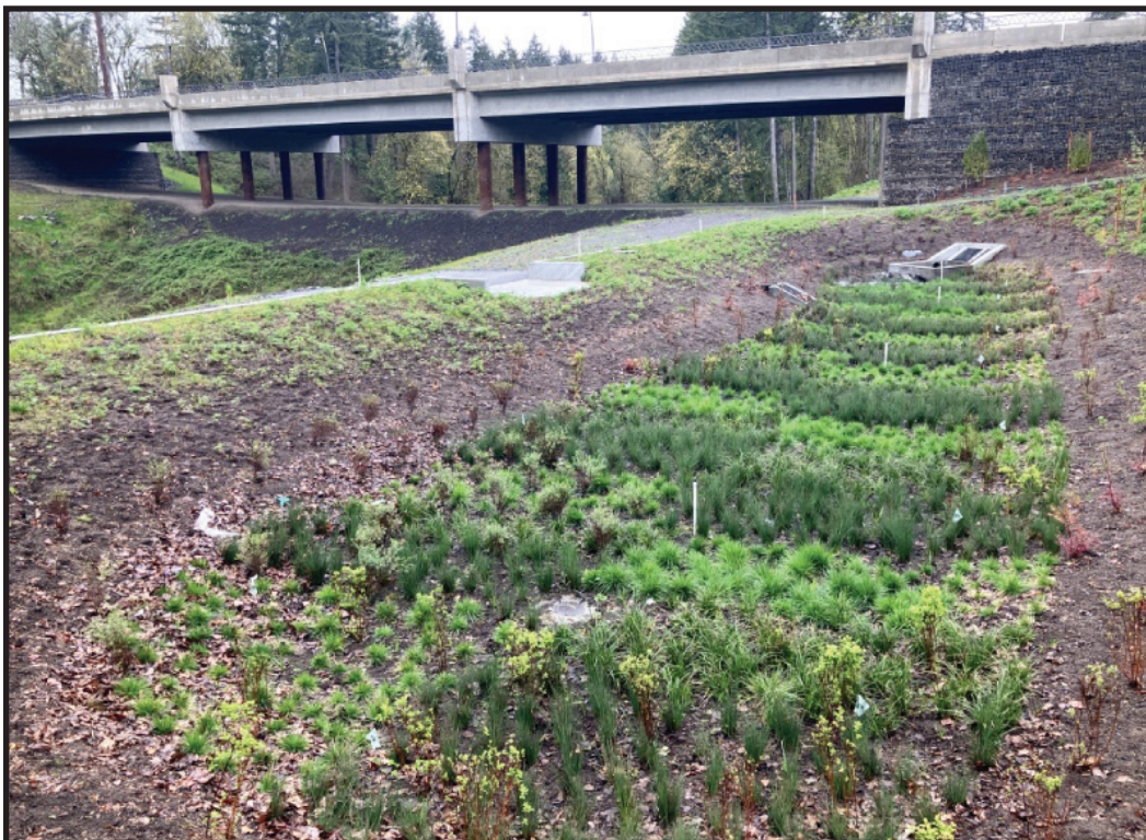
Storm Water Detention Facility at the Boeckman Road Bridge over Boeckman Creek (CIP #4212).
