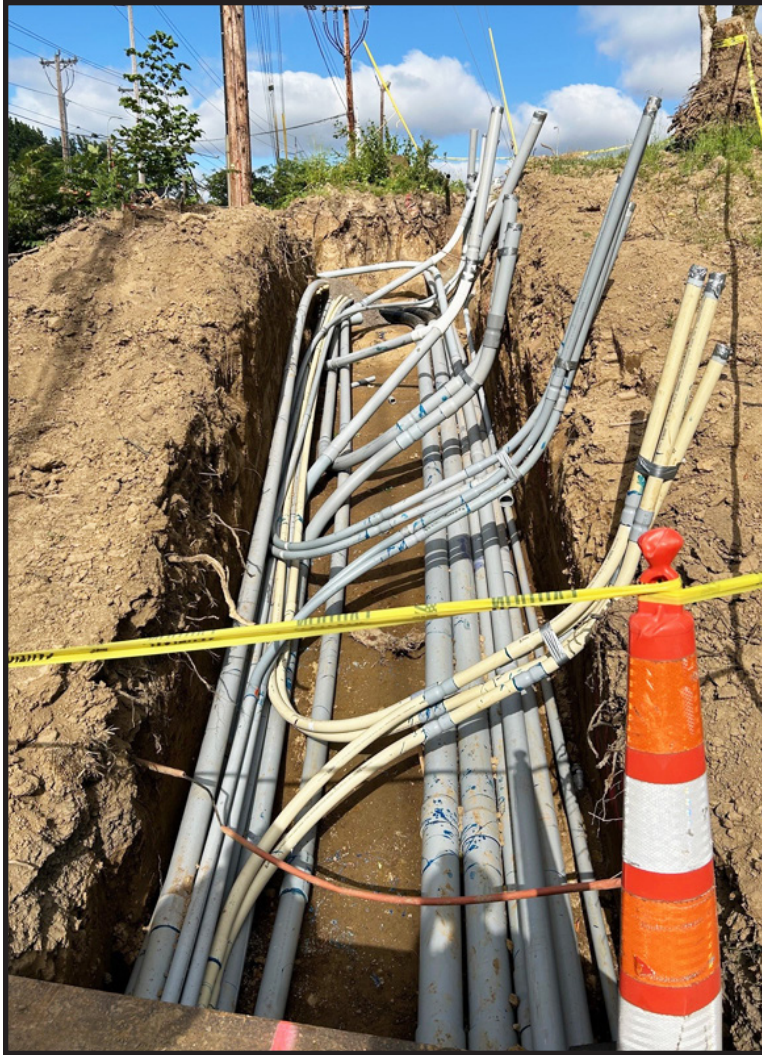
City fiber conduit in the utility trench along Boeckman road (CIP #8093).
