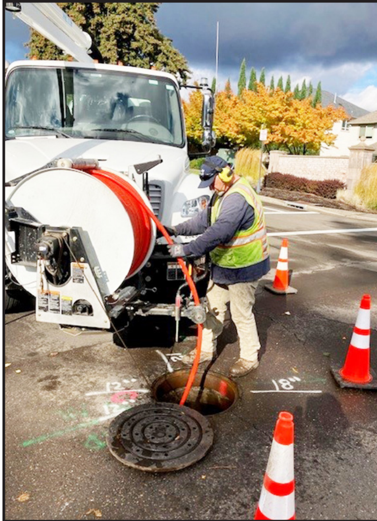
Stormwater staff performing storm system cleaning and CCTV inspection.
