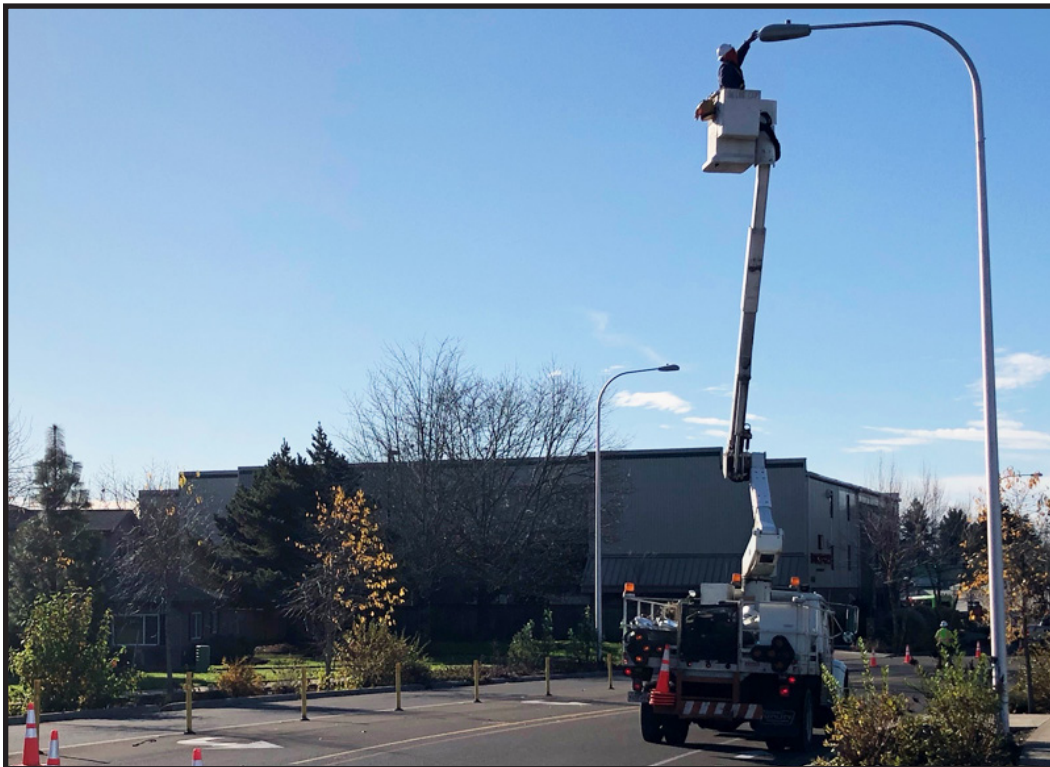
LED streetlight conversion project - light installation.
