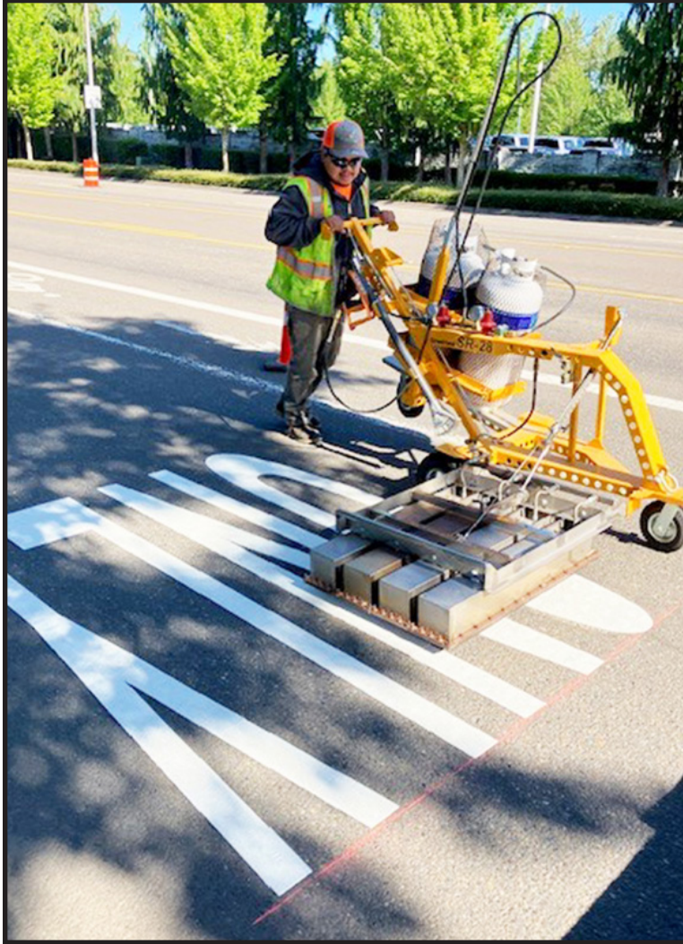
Roads staff refreshing thermal plastic pavement markings.
