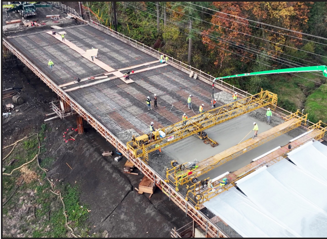
Aerial view of the concrete bridge deck pour for the Boeckman Creek bridge as part of the Boeckman Road Corridor Project (CIP #4196).
