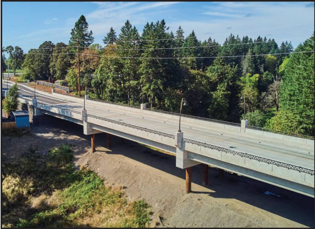
Completion of the Boeckman Road Bridge over Boeckman Creek (CIP #4212).
