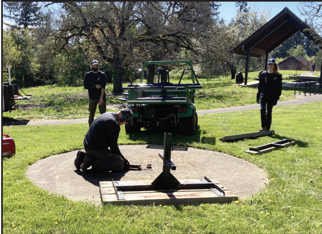
Updating picnic tables as part of the ADA park improvements (CIP #9174).
