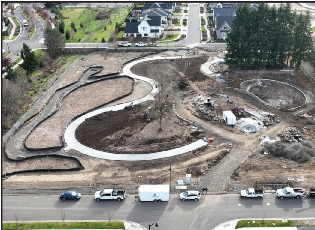
Construction of Frog Pond Neighborhood Park (CIP #9175) on January 22, 2026.
