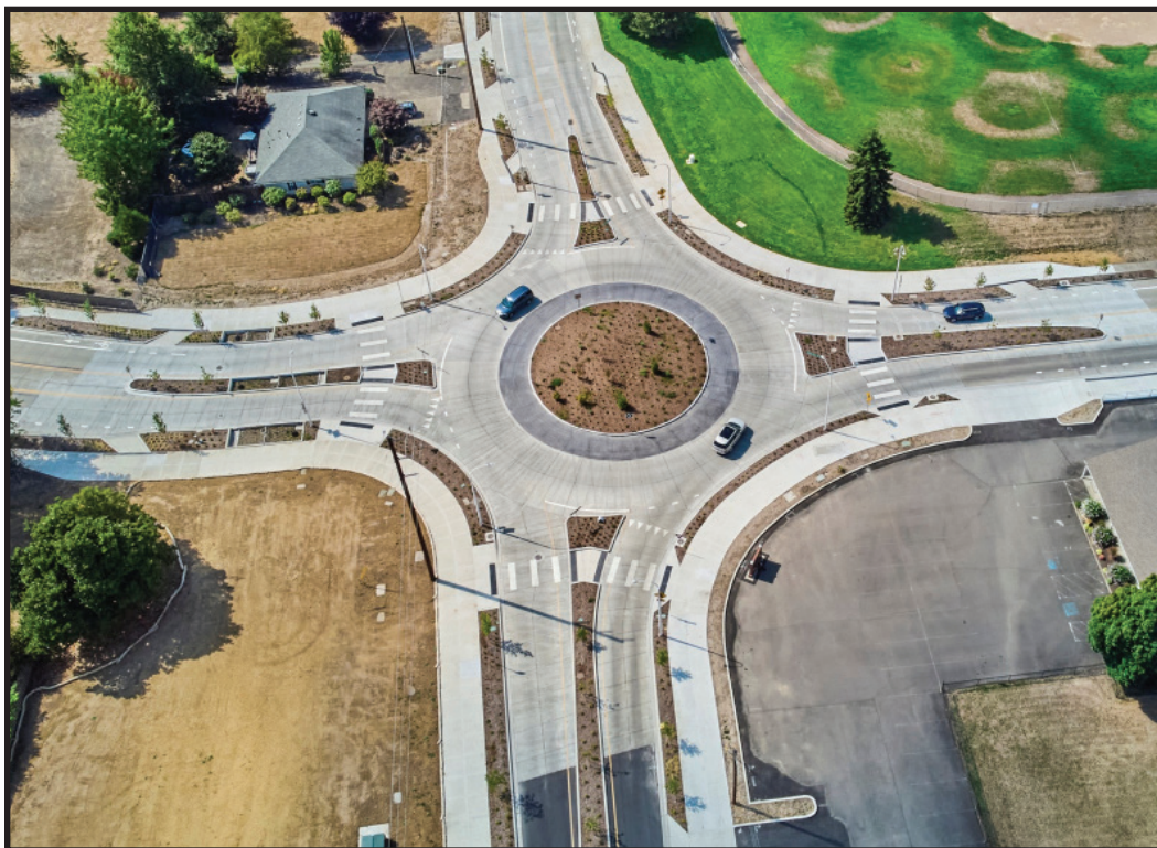
Completion of the Canyon Creek / Boeckman Roundabout (CIP #4206).
