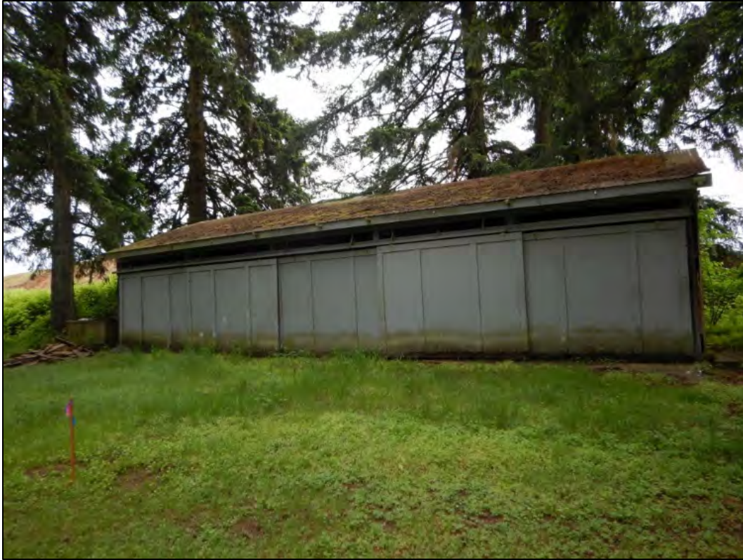
Figure 6-9. Equipment barn, looking west at the east façade.
