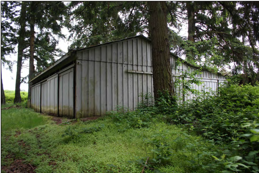
Figure 6-10. Equipment barn, looking southwest at the north and east facades.
