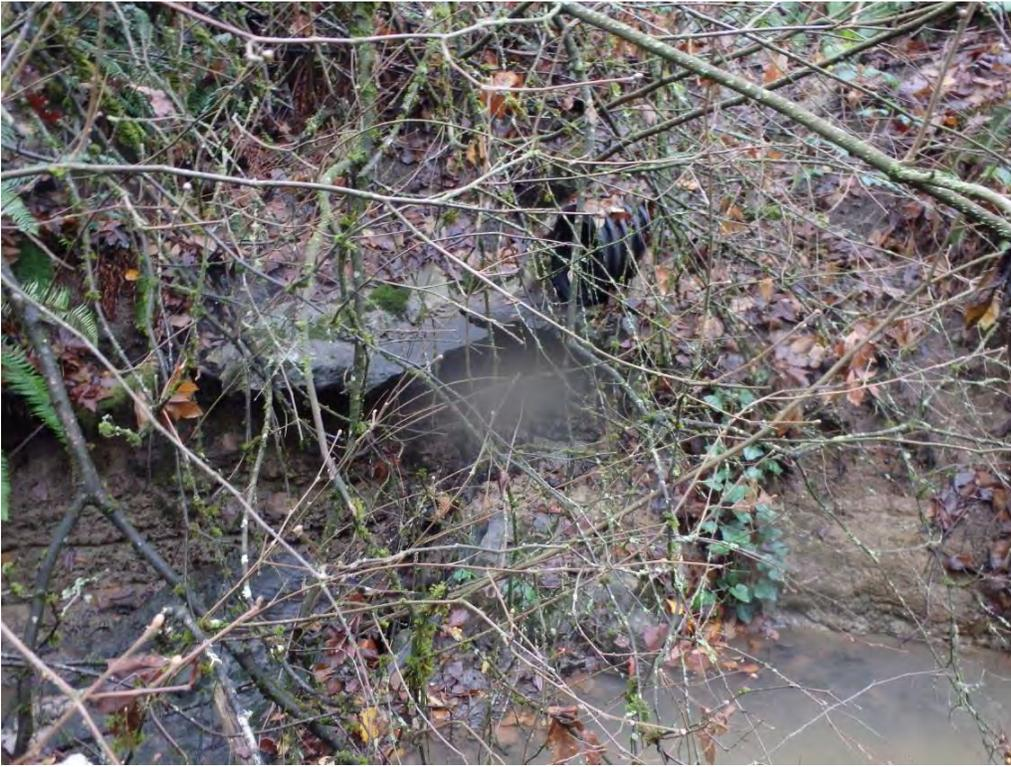
**Photo 16 Perched Culvert on Right Bank**
