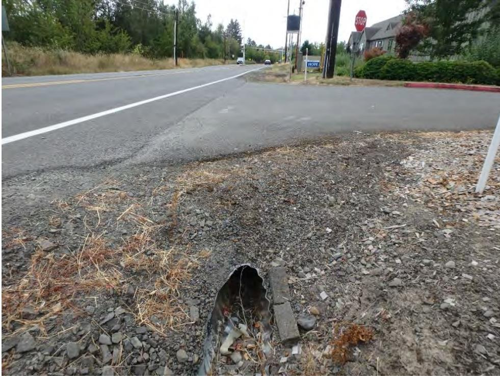
Figure 11. Pipe under church driveway is 10 inch corrugated metal at upstream end and 8 inch plastic at downstream end (Node 27).
