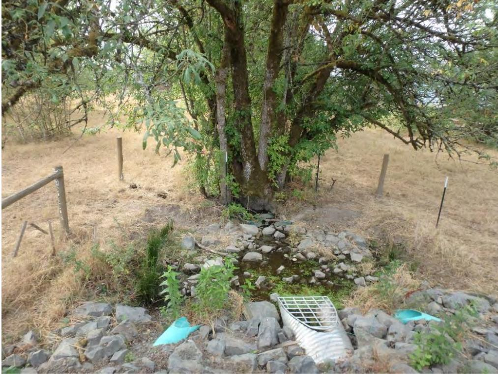
*Figure 15. Outlet of 24" Culvert south of SW Advance Rd (Node 14)*
