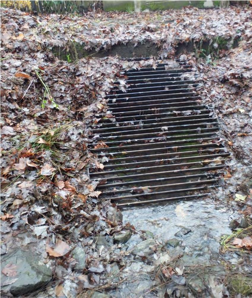
**Photo 7 36-inch culvert under SW Willow Creek Drive**
