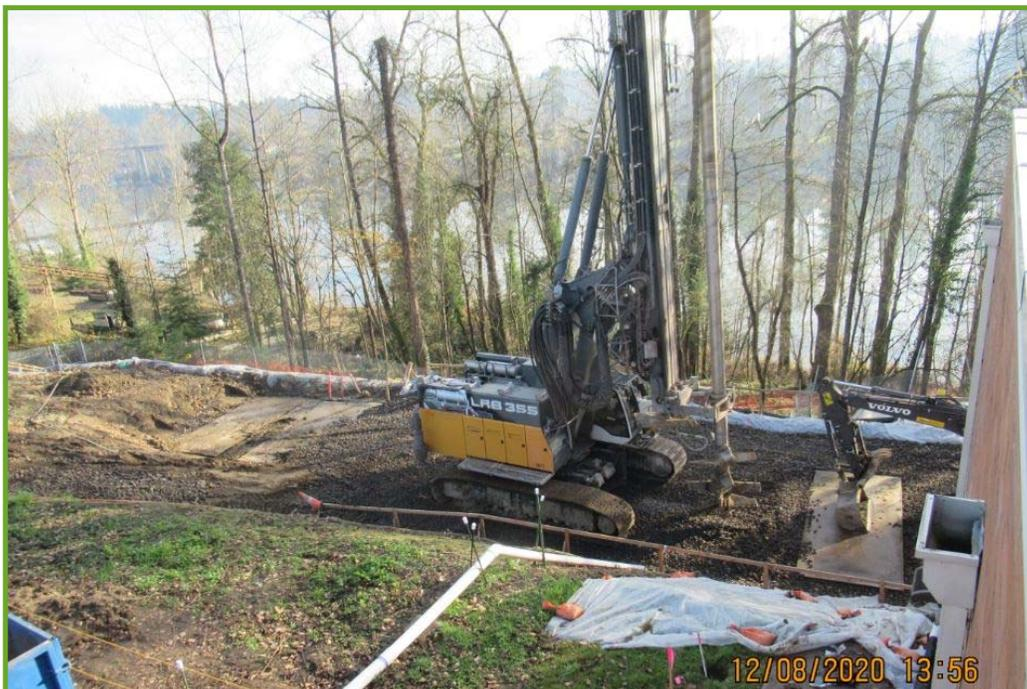
*Drill rig for deep soil mixing which will provide seismic stability of
