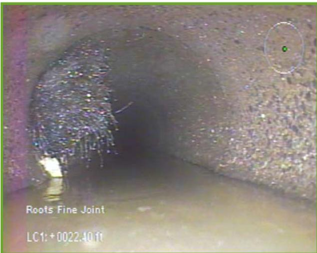
*Root intrusion into sewer pipe*
