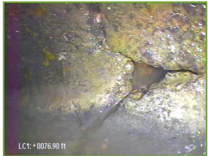
*Crack on side of sewer pipe*
