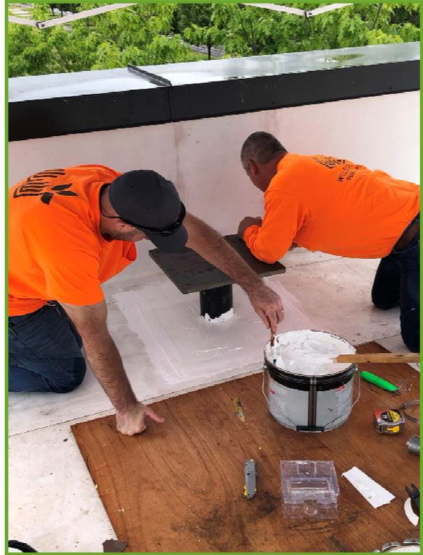
*Installation of waterproofing around the Davit Arm mounting bracket*
