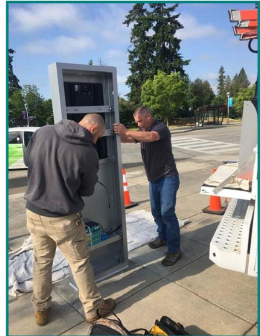
Next the solar panel had to be attached to the top of the reader board, wires inside of the unit were plugged into the appropriate terminals and the back panel was fastened to the unit with tamper proof screws. Finally, crew members called the vendor to confirm that the reader board was powered up and working properly.
