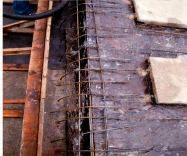
Once the repair was finished, the City's contractor, Aldercrest Construction was able to finish the staining project. The staining of the concrete was an attempt to restore the black color of the concrete so that the original design of the water feature would be reestablished. The project included cleaning of the concrete, application of two coats of stain and one coat of sealer. Notice the difference in contrast in the photos below.
