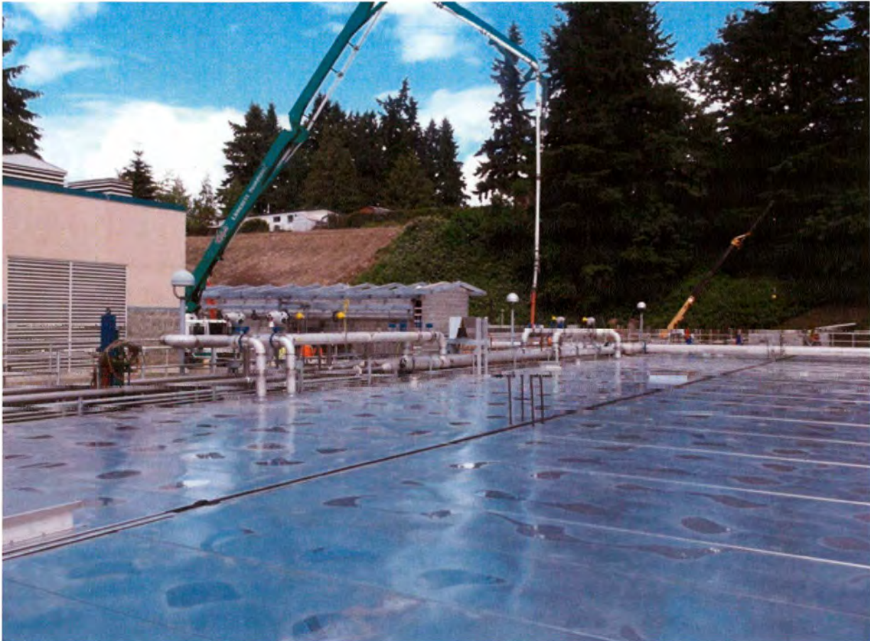
8- Concrete Pour for Selector Wall in Aeration Basin #1.
