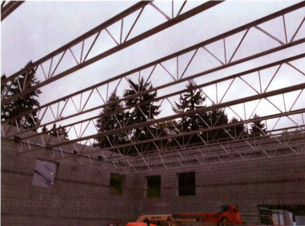
10- Roof Joists Installed at the Dewatering and Drying Building.
