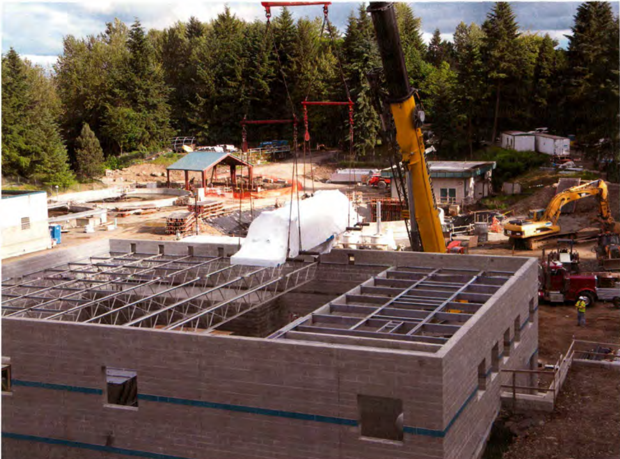
6- Installation of Biosolids Dryer.
