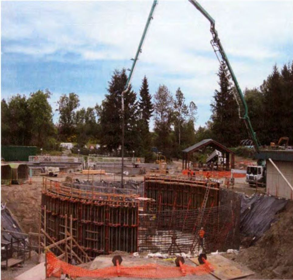
3- Secondary Clarifier #3 Wall Placement.
