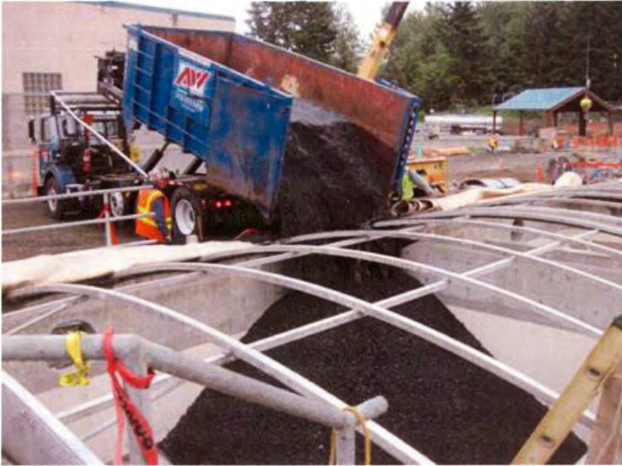
4- Biofilter Media Installation.
