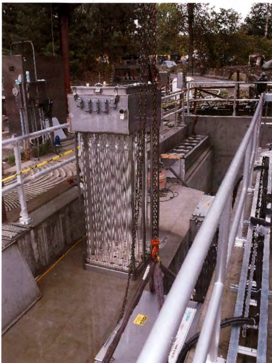
16- UV Channel and lamp module.
