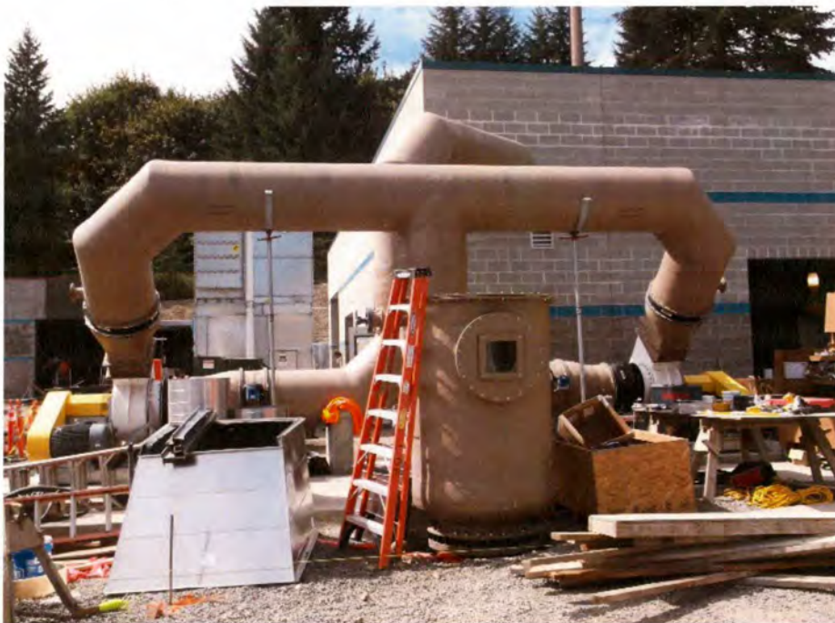
12- Foul air fans and ductwork at Dewatering and Drying Building.
