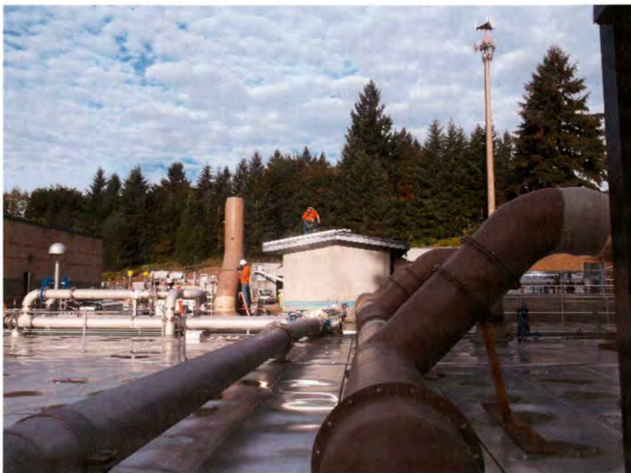
13- Foul air ductwork on Aeration Basins.
