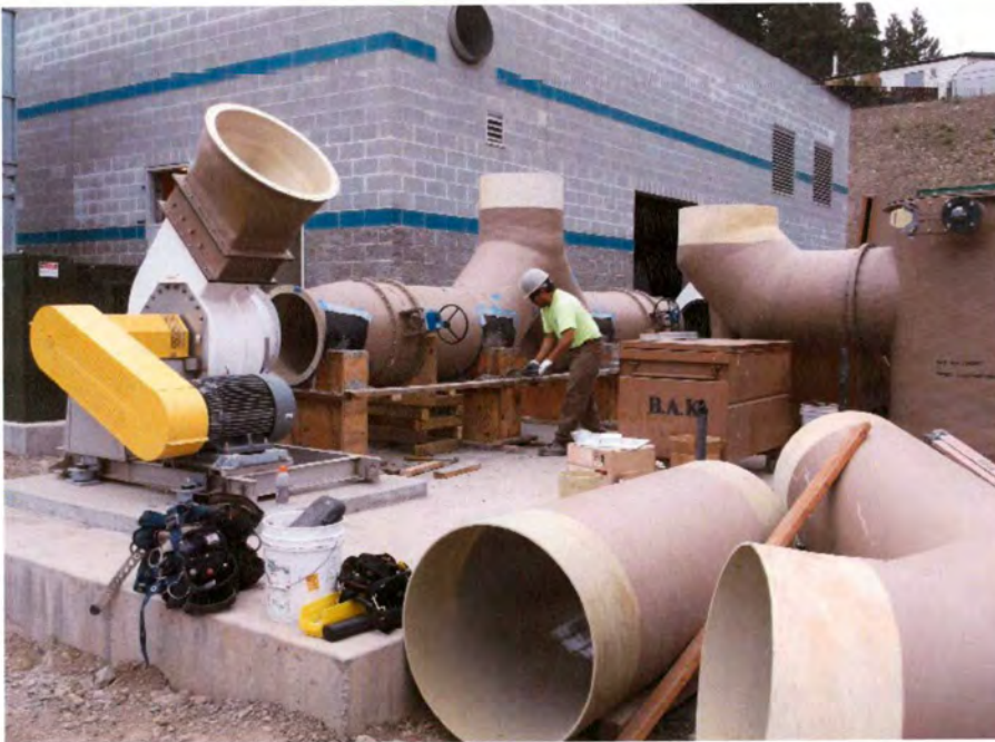
6- Foul air fans and duct at D&D Building.
