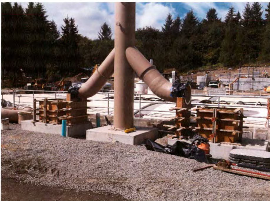
14- Foul air discharge stack at biofilter.
