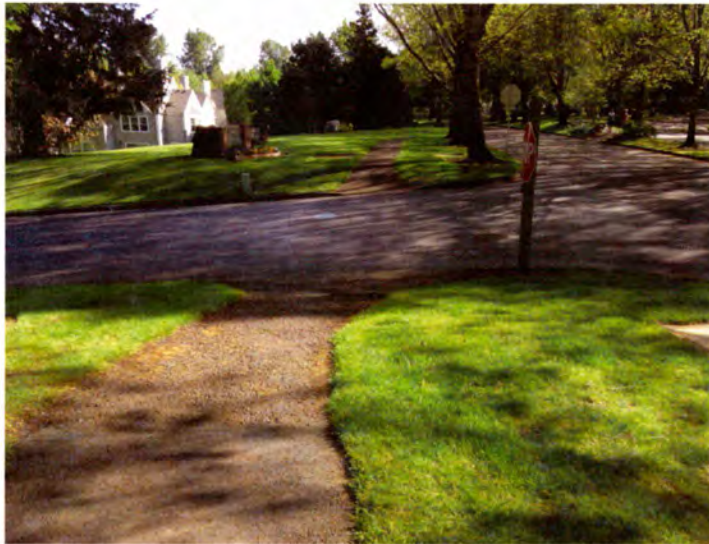
Location #5 – Surface consists of loose rock asphalt and is slippery. Install concrete ADA ramp and regrade and transition with asphalt.
