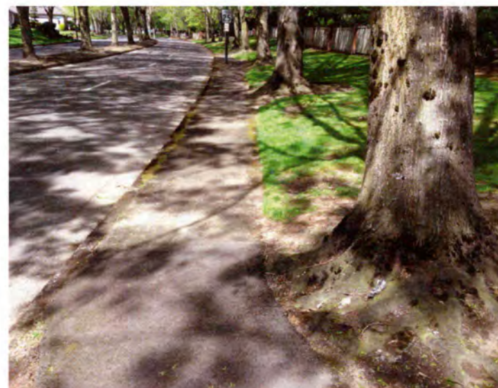
Location #17 – Tree root damage causing trip hazard at three locations. Trim roots where feasible. Regrade and repave lifted asphalt.
