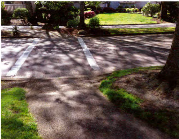
Location #7 – Tree root damage causing trip hazard. Trim roots where feasible. Install concrete ADA ramp.
