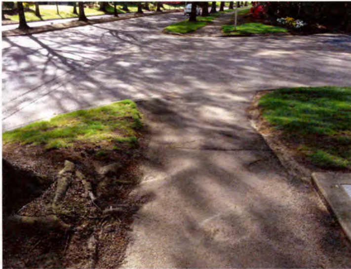
Location #1 – Tree root damage causing tripping hazard. Trim roots where feasible. Install new concrete ADA ramp.
