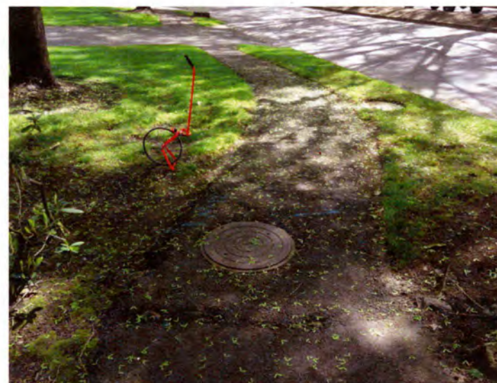
Location #15 – Poor transition to manhole lid causing trip hazard. Regrade and repave asphalt transition.
