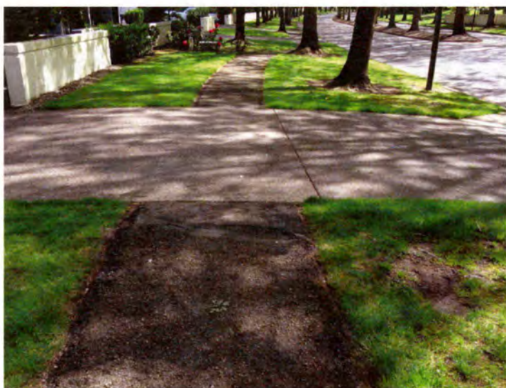
Location #14 – Poor transition to concrete driveway approach causing trip hazard. Regrade and repave asphalt transition.
