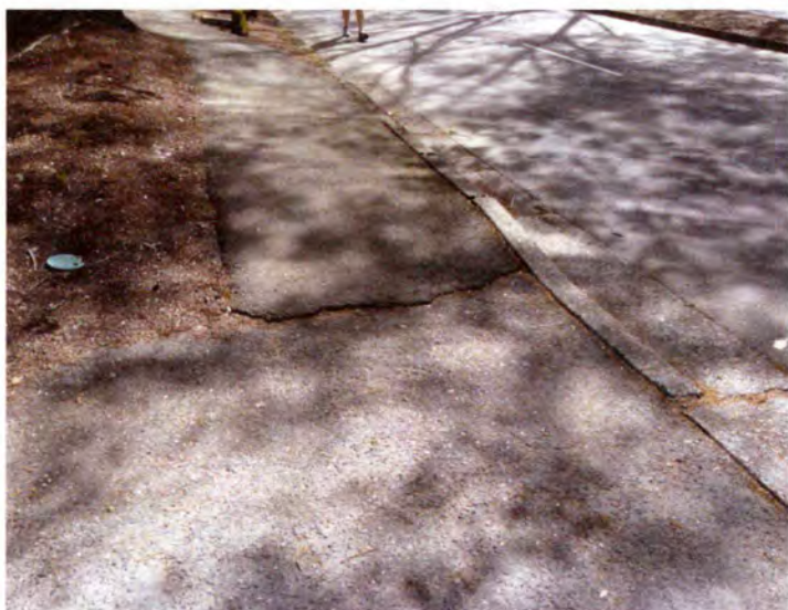
Location #16 – Poor transition to driveway approach causing trip hazard. Regrade and repave asphalt transition.
