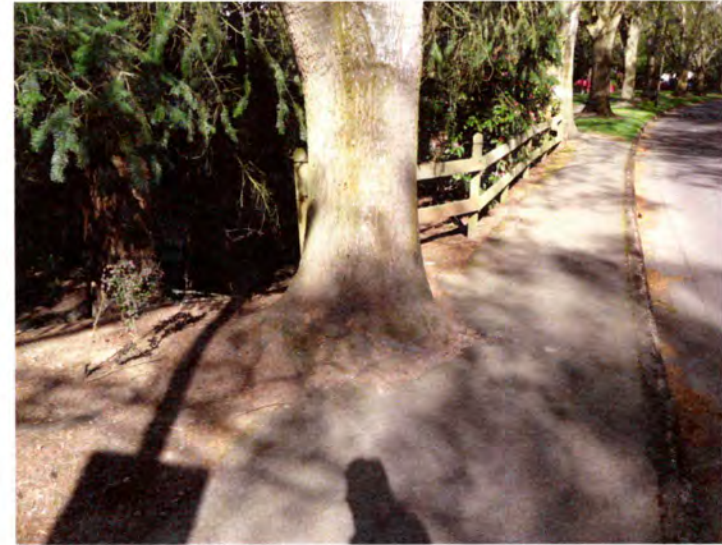
Location #2 – Tree root damage causing tripping hazard & narrow passage. Remove tree, regrade and repave lifted asphalt.
