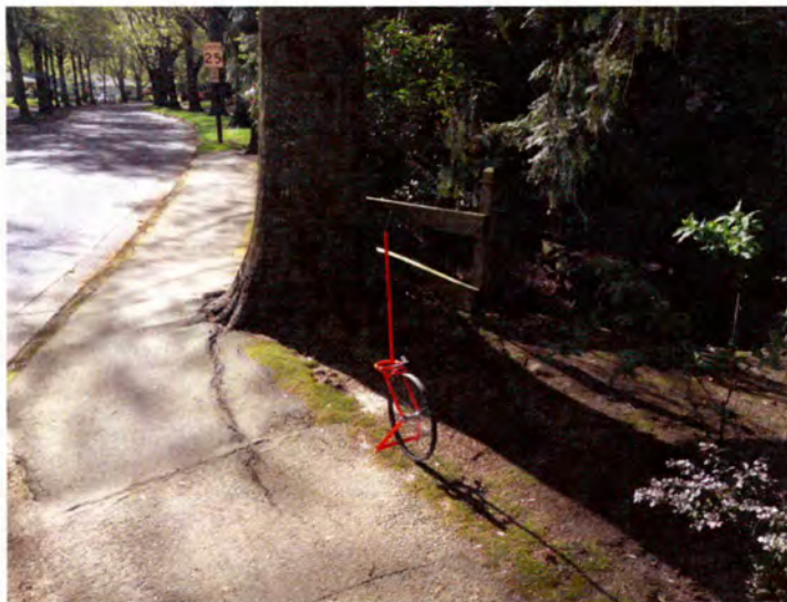
Location #3 – Tree root damage causing tripping hazard. Remove tree, regrade and repave lifted asphalt.
