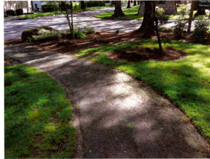
Location #11 – Alligatored asphalt causing trip hazard. Regrade and repave damaged asphalt.
