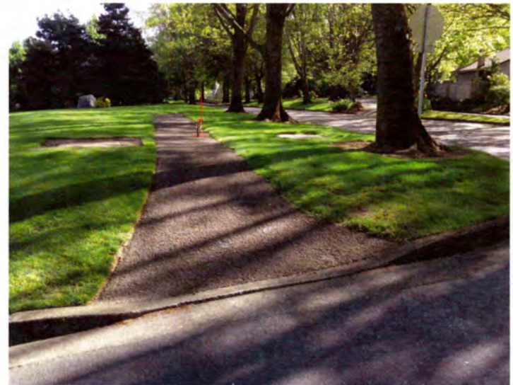
Location #6 – Surface consists of loose rock asphalt and is slippery. Install concrete ADA ramp and regrade and transition with asphalt.
