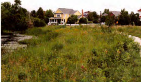
Retention Pond (Holds rainwater in wetland environment)
