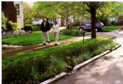
Stormwater Bioswale (Natural detention and filtration of on-street rainwater)
