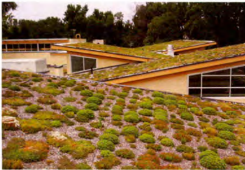
Green Roof (Reduces roof runoff and improves building insulation)
