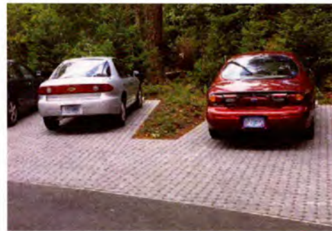
Pervious Paving (Allows rainwater to percolate into soil)
