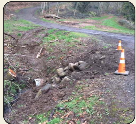
Repaired severe washout in Boeckman Creek behind the maintenance barn
