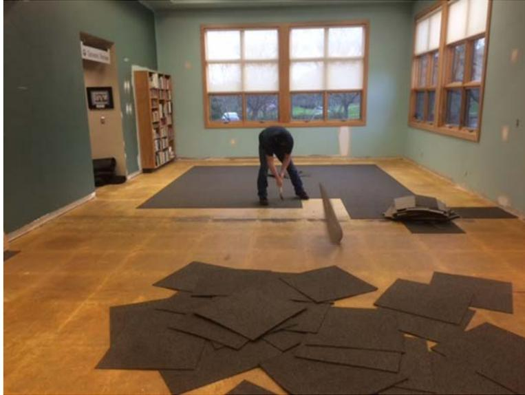
In addition to remodel, the Community Center received some sheetrock patching and new paint in the commons area, plus additional power and data cable has been added throughout. The old carpet was removed and the existing concrete slab was ground, polished, and coated with a special protective coating. Soon to come will be new carpet in the office areas and hallways.
