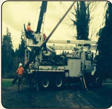
Removed overhead power lines, communication cables and poles at Duckworth Property
