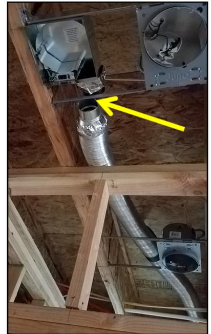
*Shown above: The bathroom exhaust duct was not fastened correctly and pulled apart. Exhaust ducts must be secured before cover with drywall.*
