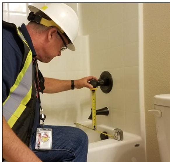
To the left is a photo of building safety inspector Mike Ditty confirming the 1-inch code required air gap on a bathtub spout during the final plumbing inspection for a new home. While not nearly as obvious to spot, air gaps are also commonly present on toilets, dishwashers, water heaters and other fixtures.
