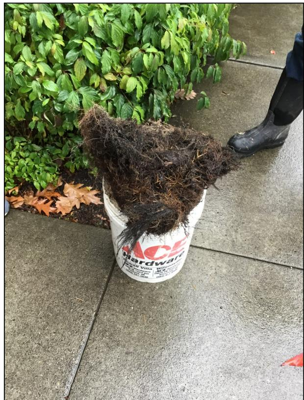
*An example of what is removed from the stormwater conveyance system. This “root monster” was pulled out of the storm line on Town Center Loop West by Public Works.*
