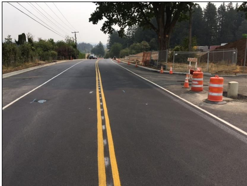
*Tooze Road—View east from the new intersection with Paris Avenue. Base lift of asphalt and temporary striping completed. Final striping will include a left-turn lane/center median here.*
