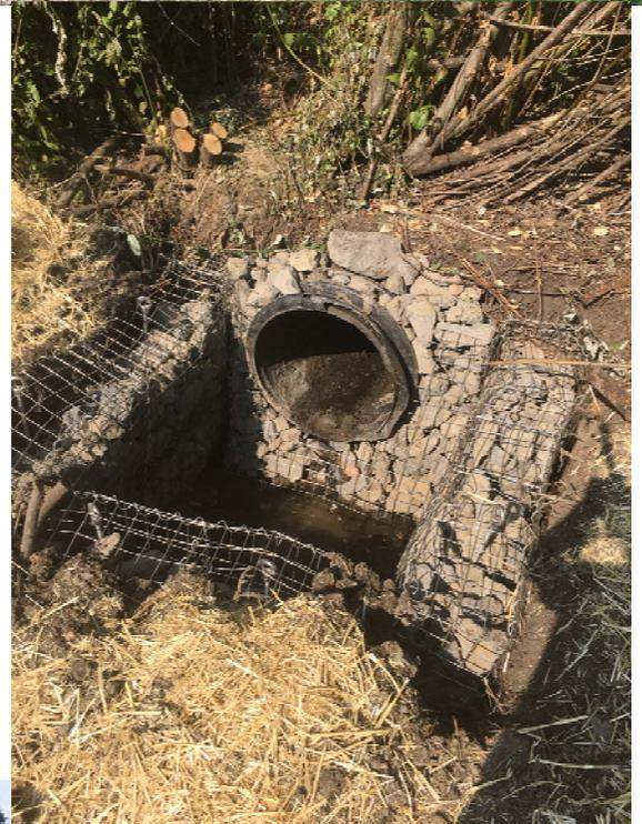
During the repairs staff was able to make some upgrades that will help the storm system better handle the flow while trapping more of the debris upstream were the debris could more easily be removed at a later date.
