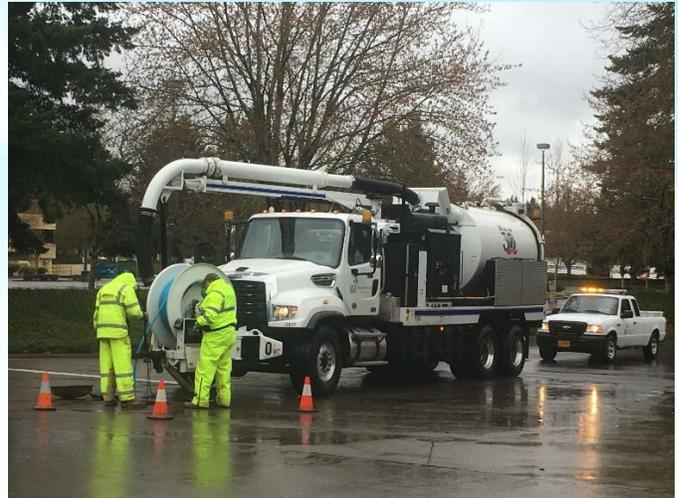
The storm water maintenance crew worked on outfall maintenance this month, including maintaining the Morey's Landing outfall at the east end of Edgewood Ct. The crew removed blackberries and other vegetation, trash and woody debris from the outfall channel. The sewer crew also maintained the water quality manhole just upstream of the outfall structure.
