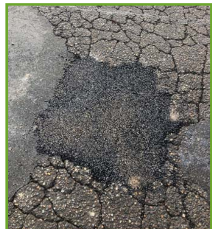
Sealed pothole
