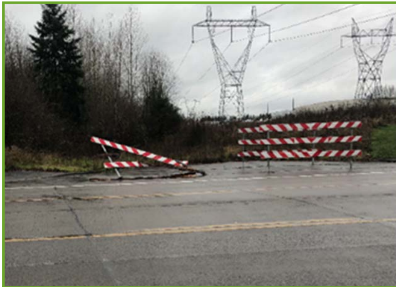
Severely damaged barricade
