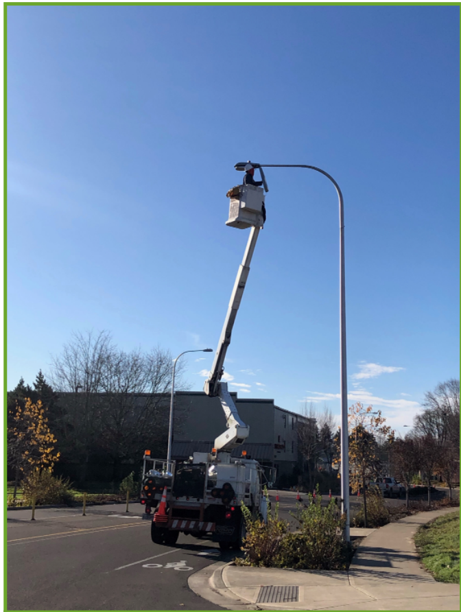
Changing streetlight from HPS to LED
