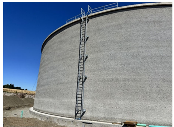
Reservoir access ladder installed
