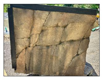
A shotcrete "rock face" wall is being installed at the east side of the trail under the bridge (left). The shotcrete is hand carved to resemble a rock face (right). The test panel is 6 feet tall.
