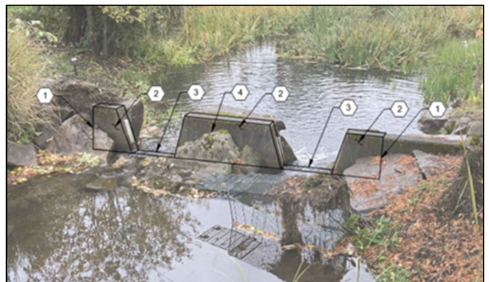
A flow weir structure shown above will need modified as a part of the project.
